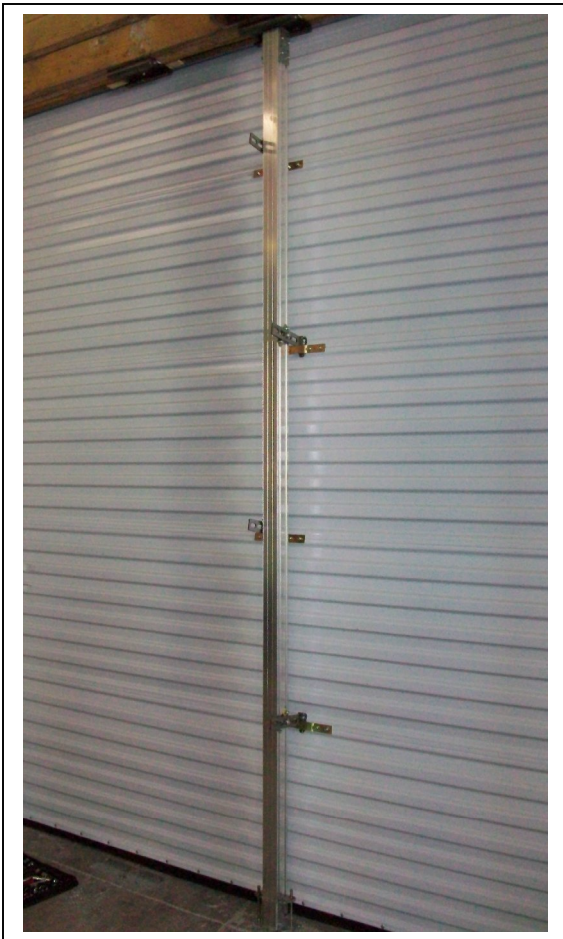
Picture of Installed brace on a door
